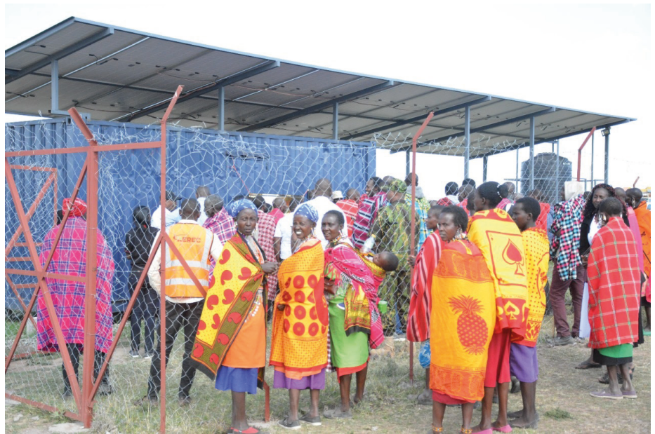
Members of the Olderkesi community at the Olderkesi mini grid
